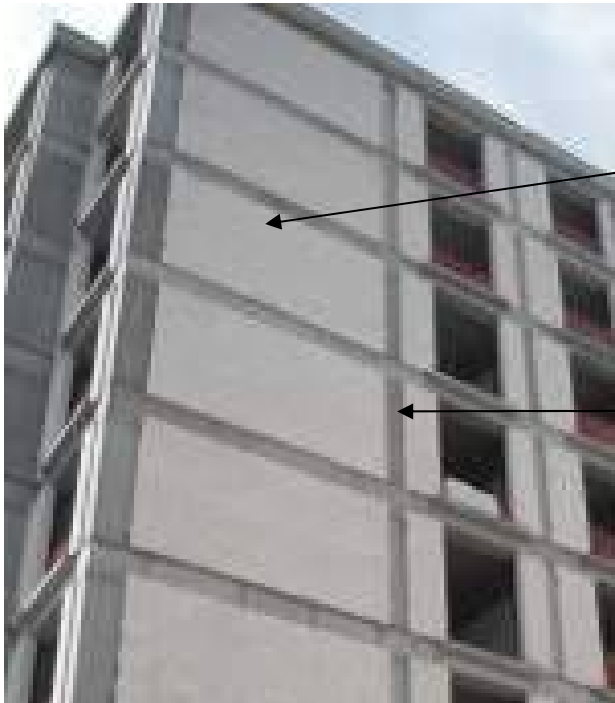
a) Prior to insulation with Ytong Multipor
