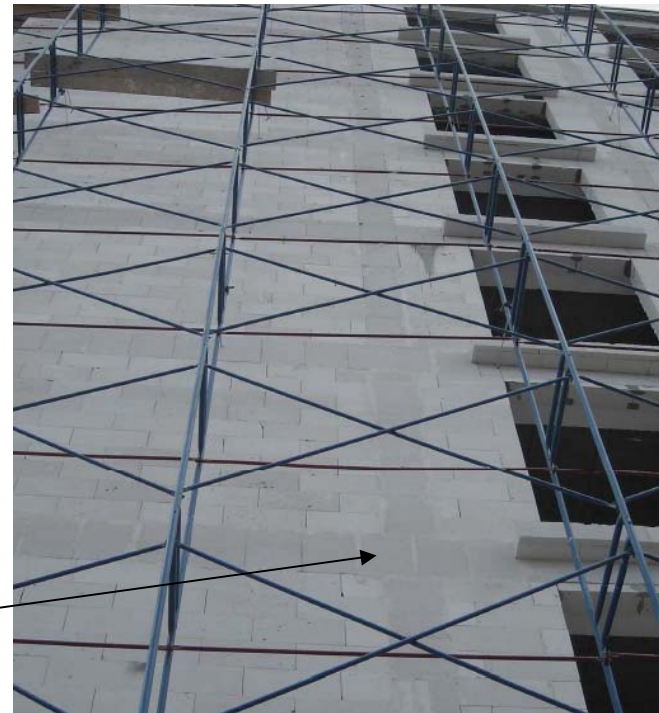
b) After insulation with Ytong Multipor
